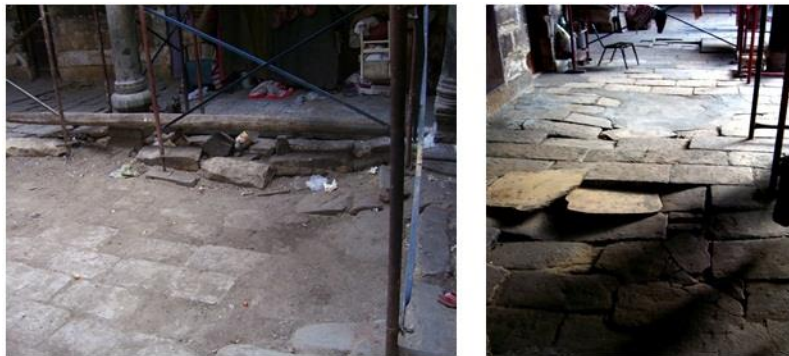
Figure 11: soil settlements
